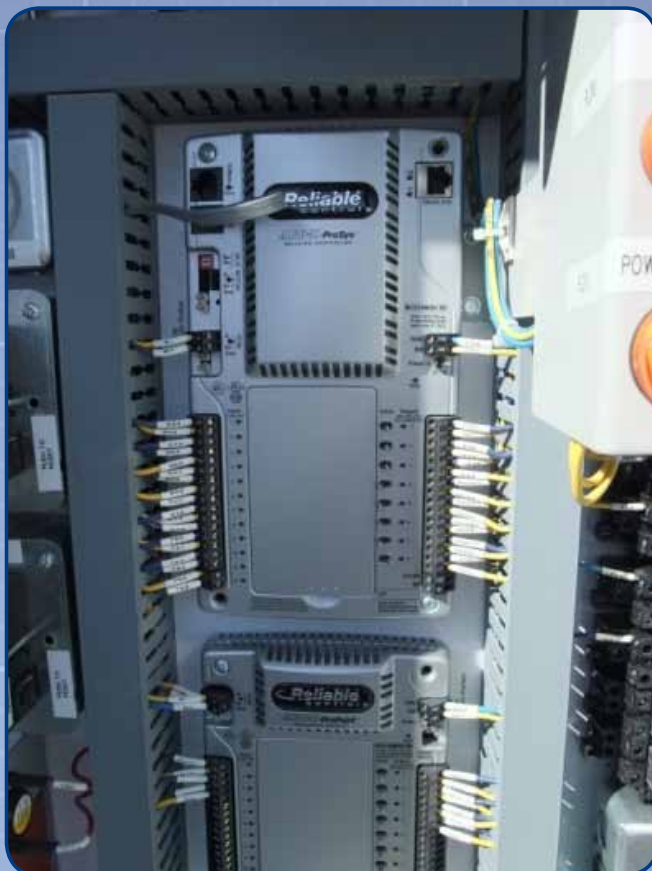
Programmable Logic Controllers by Reliable and Rockwell Automation provide ultimate unit control
