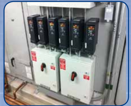
Factory mounted controls and interface from AHU to DDC system
