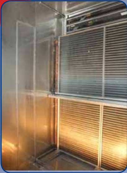
Wash down Inner liner
