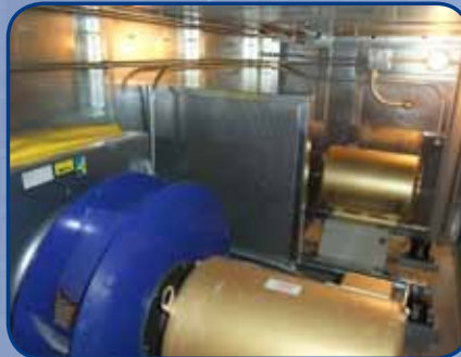
Direct Drive Plenum Fans save energy and eliminate maintenance needed with belt drive fans
