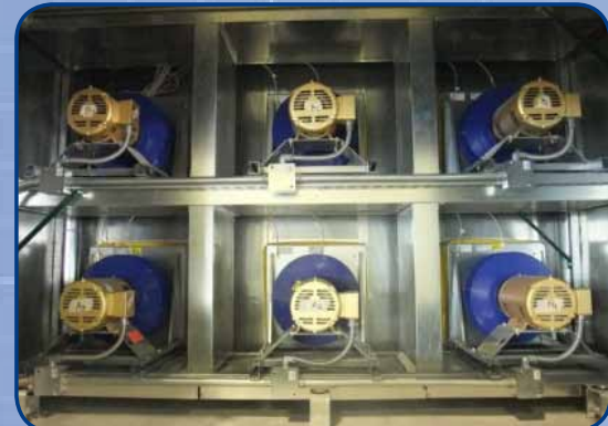
Multiple fan array application conserves unit length
