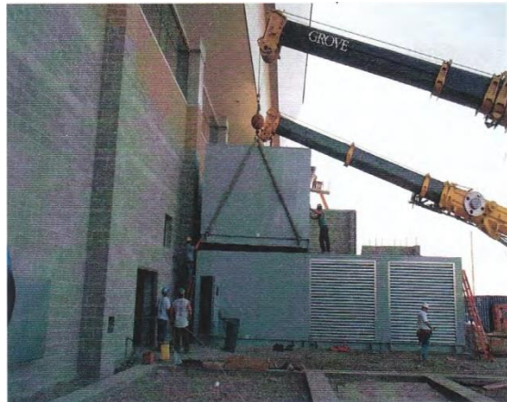
Two 25 ton cranes required for a 75-foot reach
